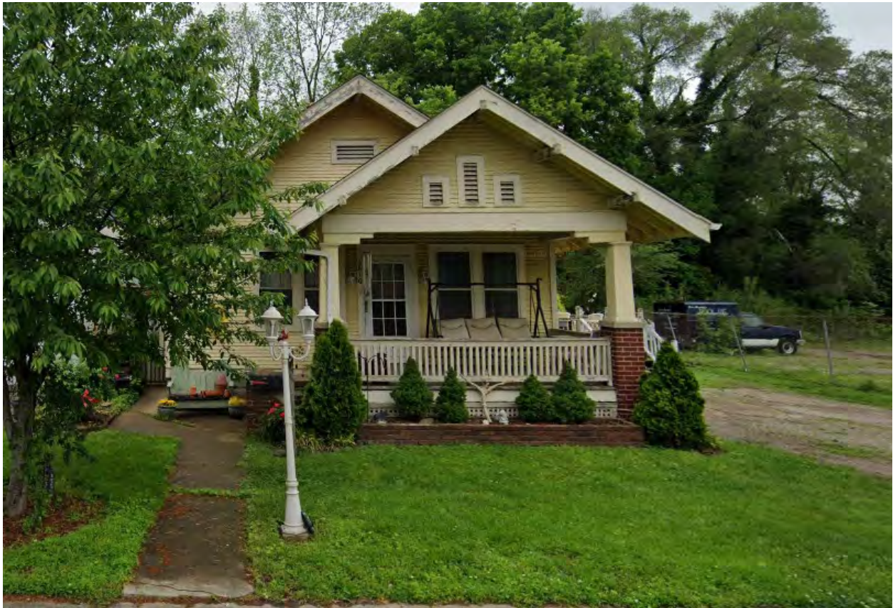
Figure 6: Imogene Whitley House, 6810 Main Street
